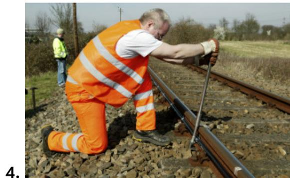
DuoTrack® is an innovative all-in-one system solution for quick, cost-effective and long-term railway cabling for non-electrified regional railway lines. Top left: the DuoTrack® cable; bottom left: laying the cable using the special vehicle; bottom right: attaching the cable with special holding clamps produced by Contec; top right: the laid cable.
