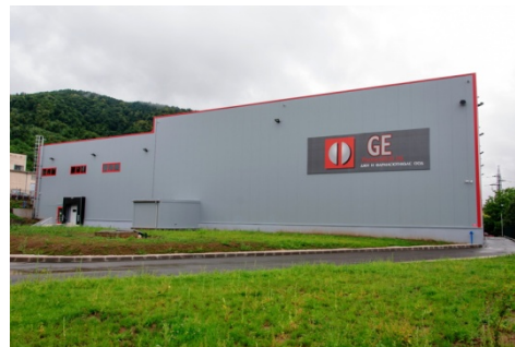
Plant 2 in Botevgrad – Beginning of production in 2016
