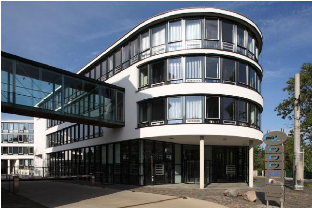
The Markkleeberg location of enviaM (photo credit: enviaM)
